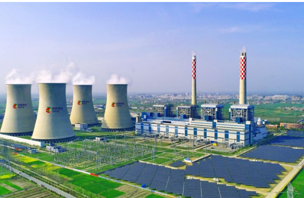
国家电投集团上海电力田集发电厂 SPIC Shanghai Electric Power Tianji Power Plant
