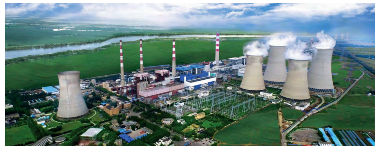
国家电投安徽平圩电厂 SPIC Pingwei Power Plant in Anhui
