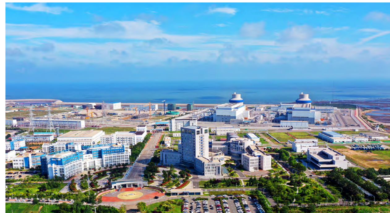
国家电投山东海阳核电一期工程 1、2 号机组 Units 1 and 2 in the Phase I Project of SPIC Haiyang Nuclear Power Plant in Shandong
